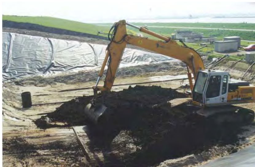
Figure 4-45. Construction of the Nauerna pilot-scale landfill (van Zomeren and van der Sloot, 2006b).
